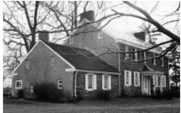
The original Vanhorn house built c. 1740's at left. The right window was the door. Richard Leedom added the larger, north side addition in 1779. The house was later in the Luff family and is now the home of Scott and Dianne Thomas.
