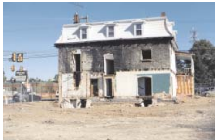
The back of the Spread Eagle Inn, stripped of it's newer additions, awaits preparation for its move about 20 feet to the right and towards you in this picture.
